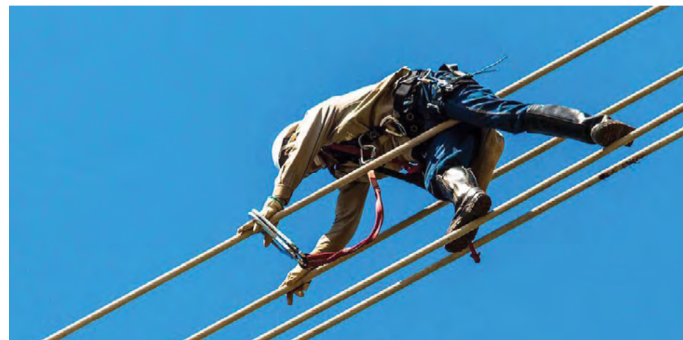
Transmission Line Maintenance.
