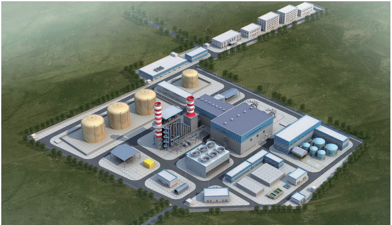
中国信保承保的孟加拉迈门兴360MW双燃料联合循环电站项目 Mymensingh 360MW Dual-fuel Combined Cycle Power Plant Project underwritten by SINOSURE
