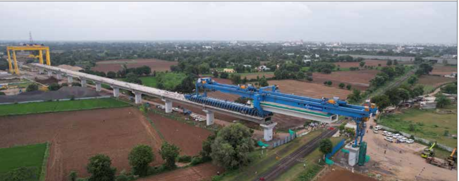
Indigenously designed and manufactured Full Span Launching Machines for Mumbai-Ahmedabad High-Speed Rail (MAHSR)
