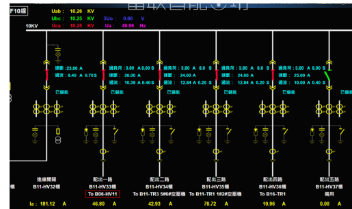
Power Monitoring Screen
