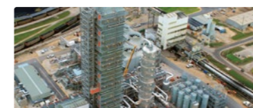
CO 2 recovery plant in the US
