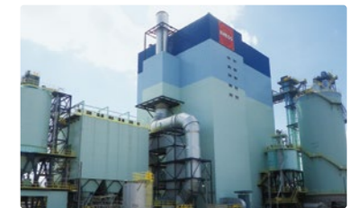
Muroan Biomass Power Plant
