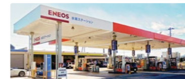
Hydrogen station (integrated into service station)
