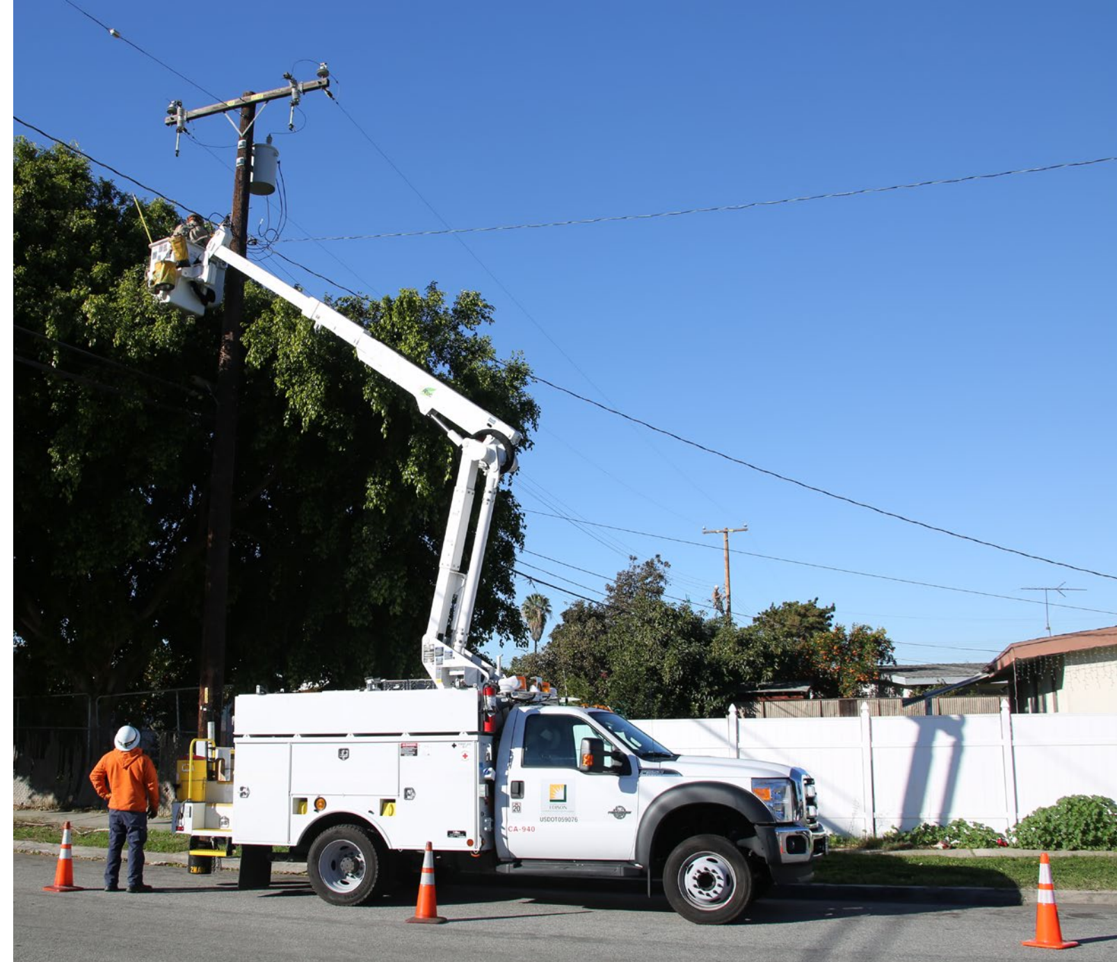
SCE is installing electric power takeoff systems on its fleet of bucket trucks.
