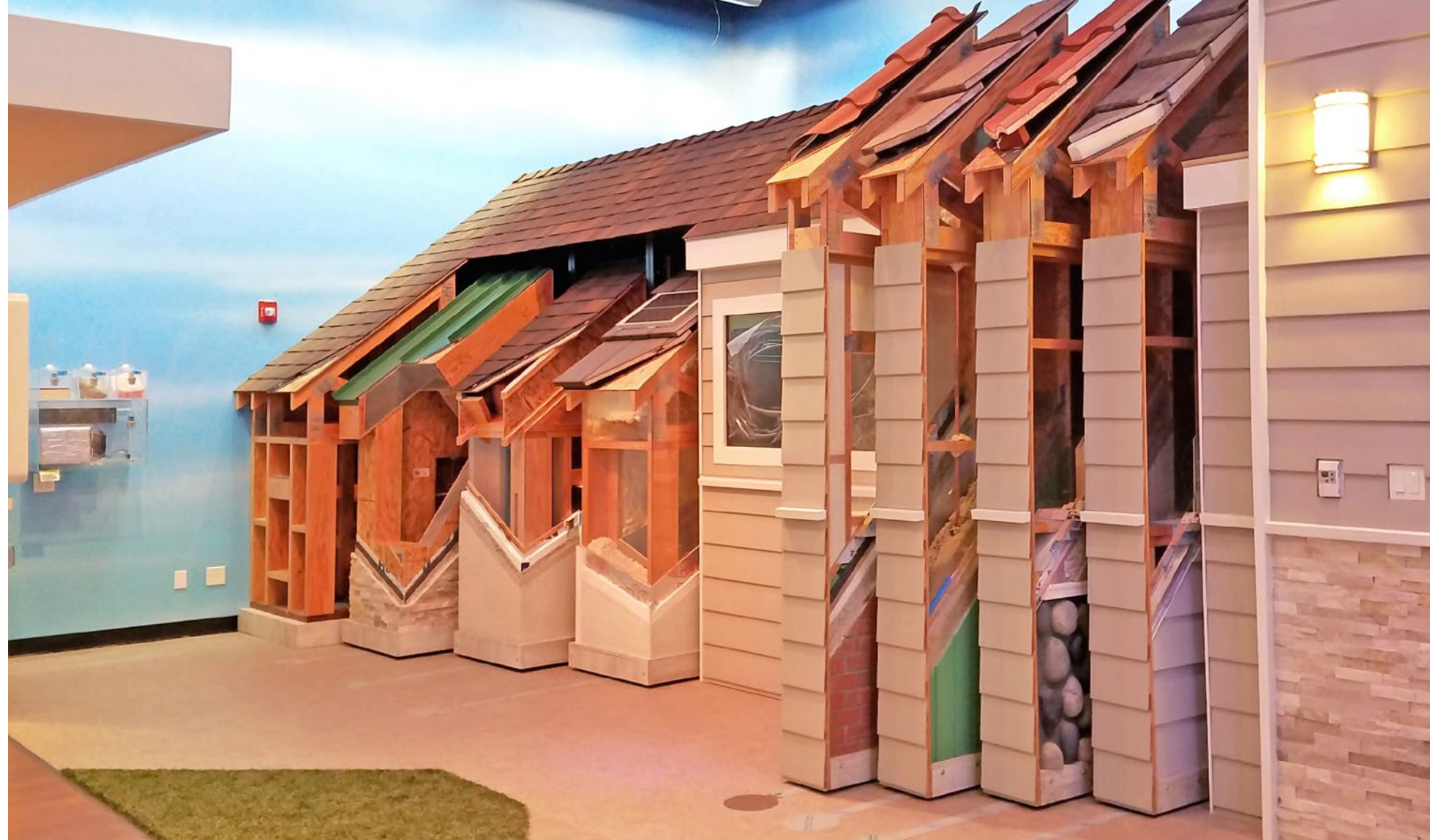
A new interactive display at SCE's Energy Education Center teaches customers about high performance building envelopes, a major part of a ZNE home.
