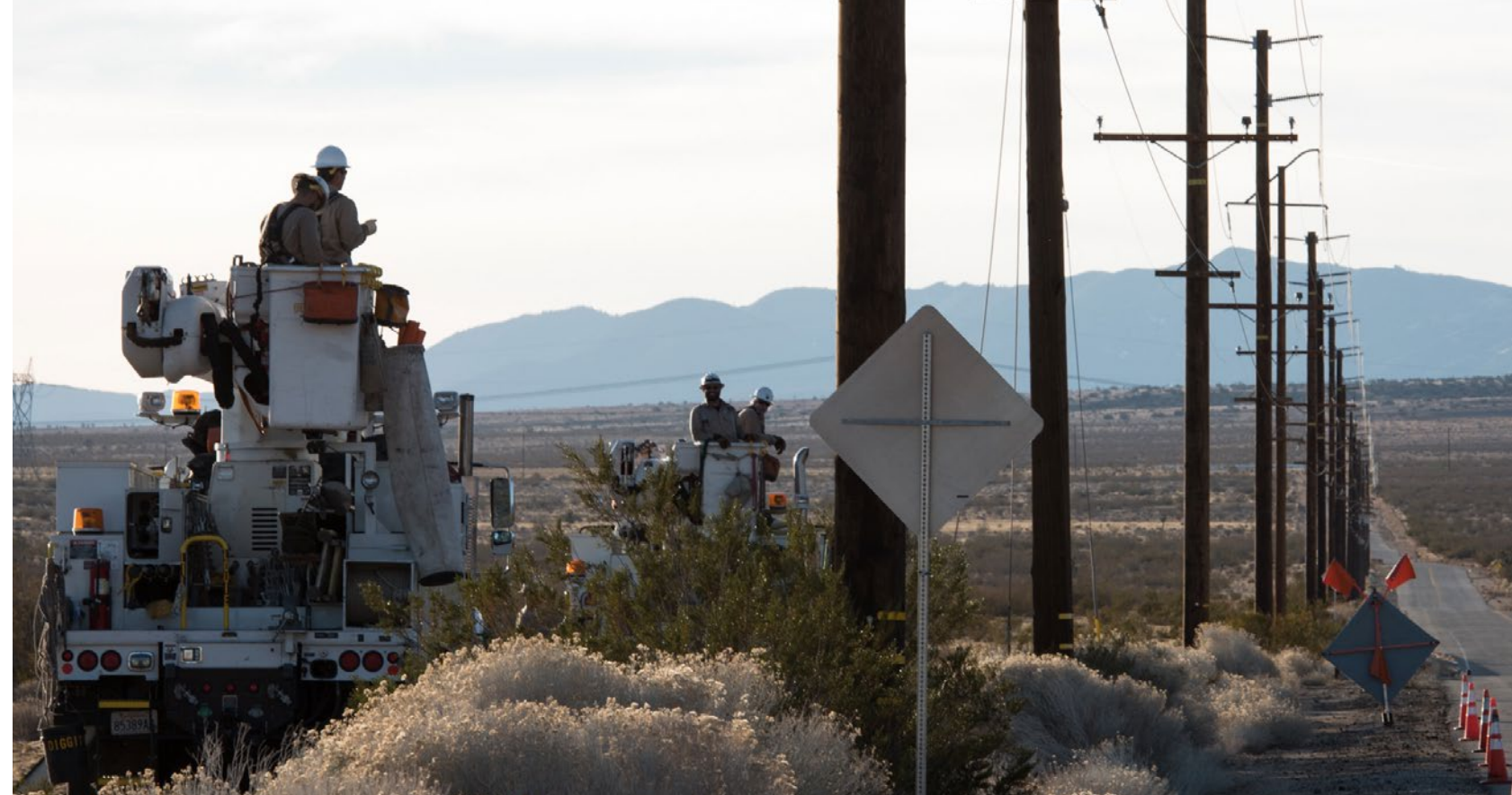
SCE workers perform system improvements to strengthen the grid.
