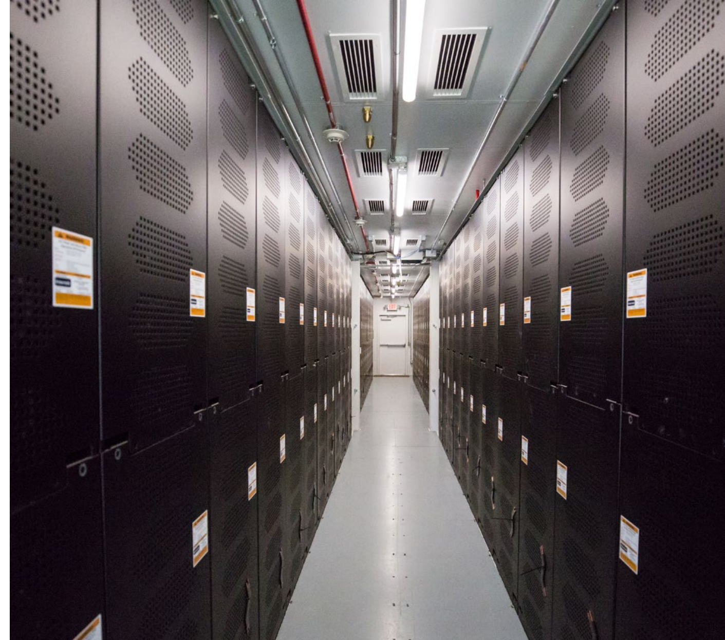
Lithium-ion batteries operating as part of the Hybrid Enhanced Gas Turbine system at the Center Peaker Plant in Norwalk, California.
