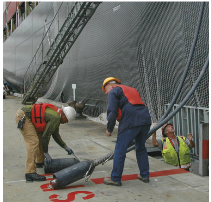
A container vessel plugs into shoreside electricity at the Port of Oakland.
