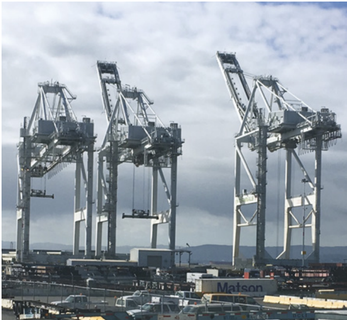
Raised SSA cranes at the Port of Oakland.
