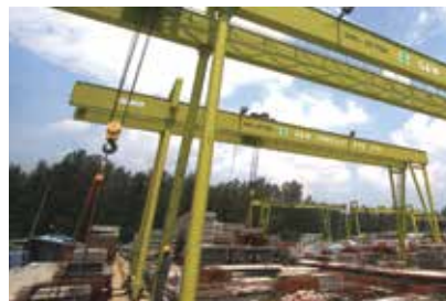
▲ G&W Precast Yard
