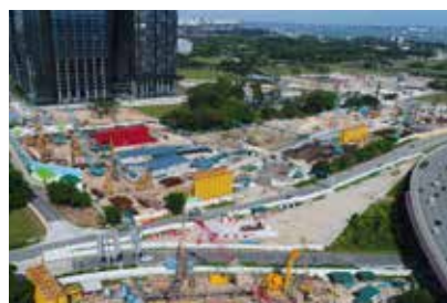
▲ Marina Bay Cut & Cover Tunnels
