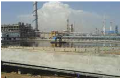
▲ Bertam DAF Water Treatment Plant (Melaka)
