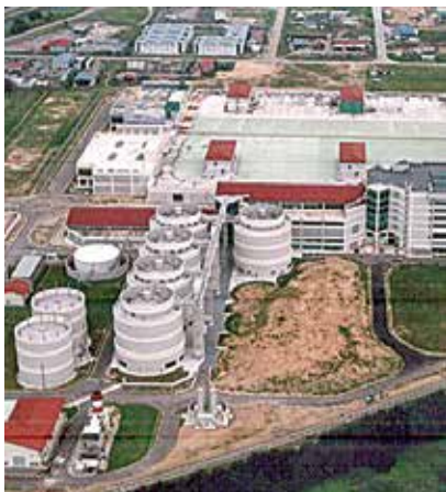
▲ Changi Water Reclamation Plant
