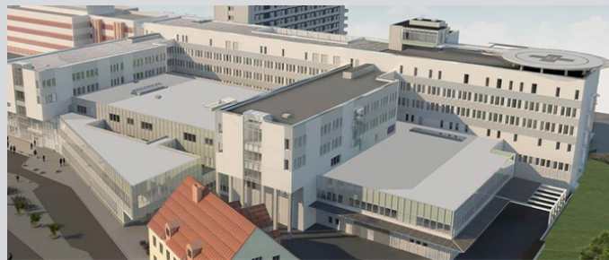
Eskilstuna Hospital construction site
