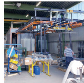
After the switch to LED lighting
