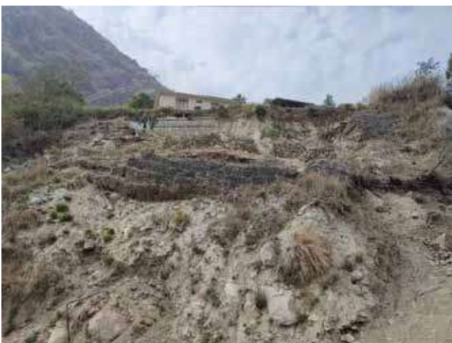
Landslide Before Protection
