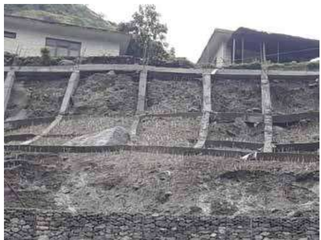
After Landslide Protection
