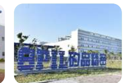
Zhong Ke Facility II
